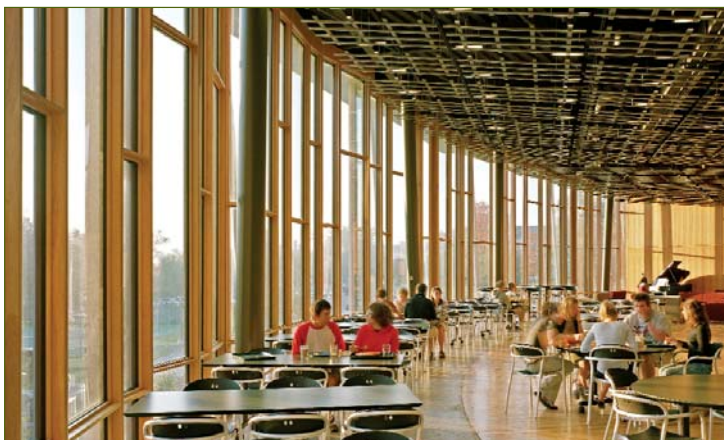
Atwater Commons dining hall floor at Middlebury College in Vermont is 6,500 square feet of hard maple, entirely harvested from campus-owned forests. Serving 700-900 students daily, the floor holds up well. Once yearly, it is buffed down to the bare wood and a low-VOC, water-based sealer is applied.
